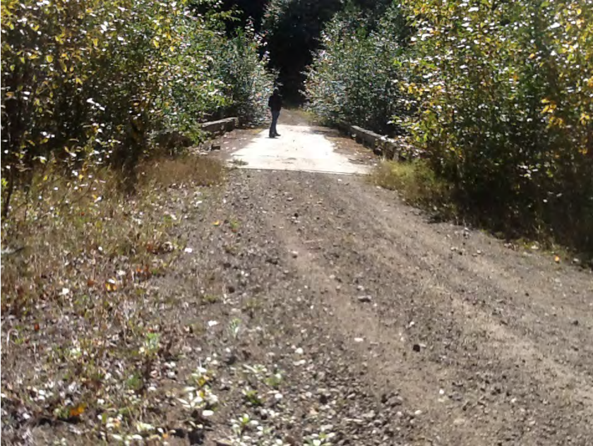
Right approach facing structure
