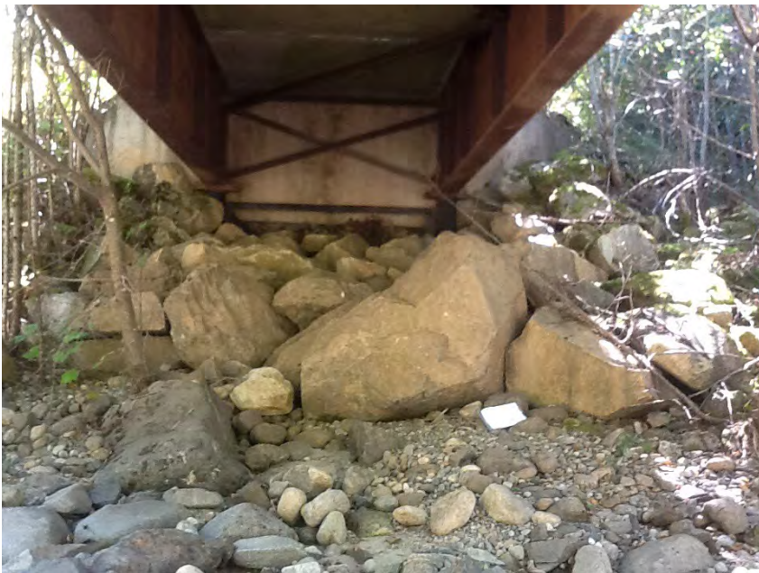
Left Bank Abutment when facing downstream
