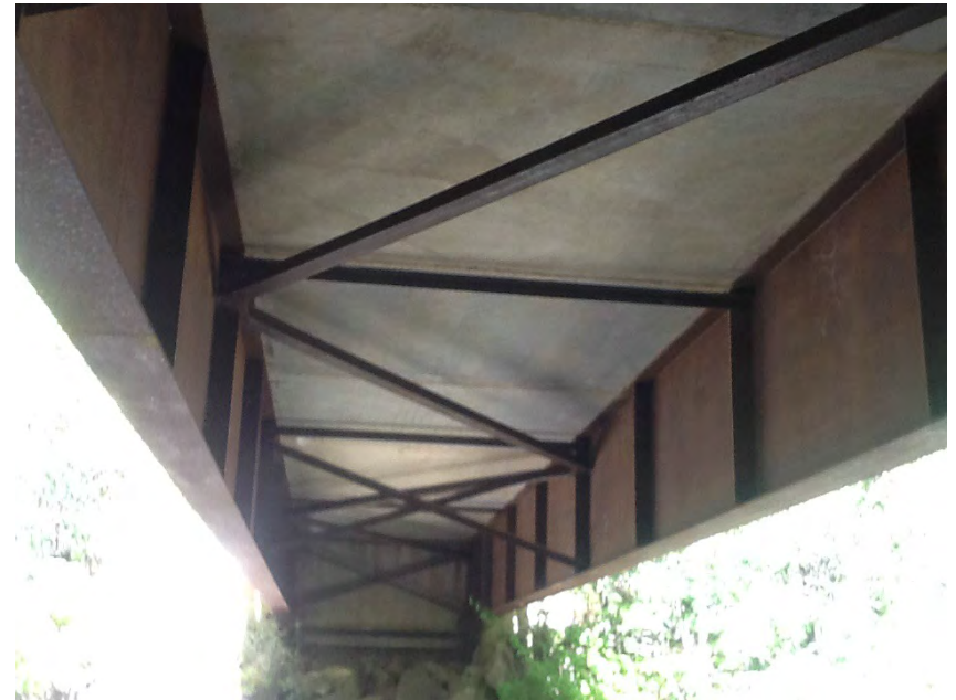
Underside of bridge
