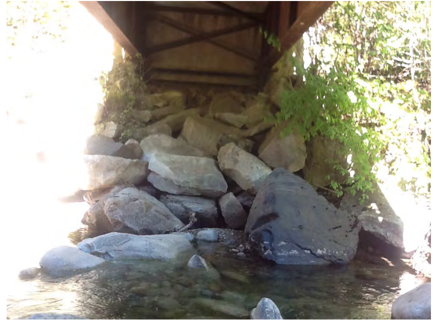
Right Bank Abutment when facing downstream
