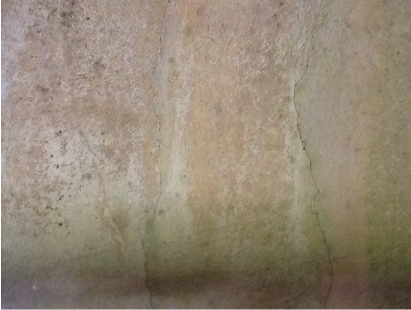
Right Bank Abutment when facing downstream
