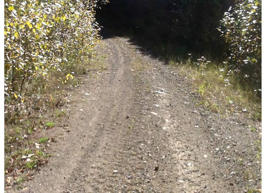
Left approach facing away from structure
